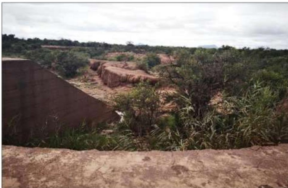
**Figure 4-30** View of the erosion gully downstream of a weir
