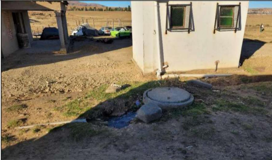
**Figure 4-69** Surcharging manhole with the sewage being directed towards the wetland.
