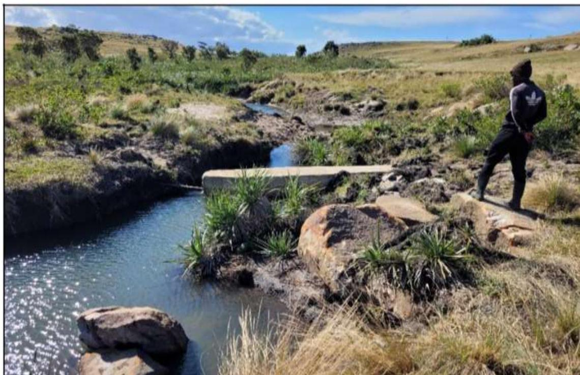
**Figure 4-89** Xolobeni wetland: Eroded palmiet wetland upstream of the water supply pipeline crossing point. Portions of the pipeline has been encased in concrete, however the channel has bypassed the concrete and has exposed portions of the pipeline
