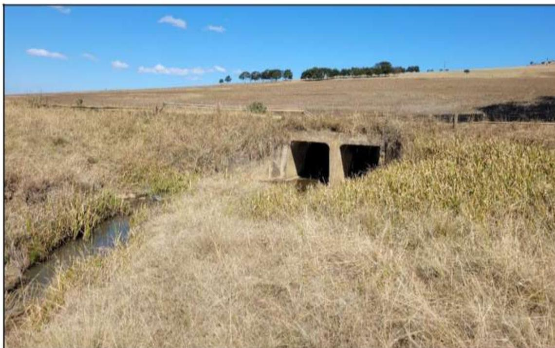
**Figure 4-100** View of the road culvert associated with the R61 which has led to the formation of a small headcut erosional feature upstream of the culvert. The headcut has not progressed too far due to the shallow bedrock layer within the system.
