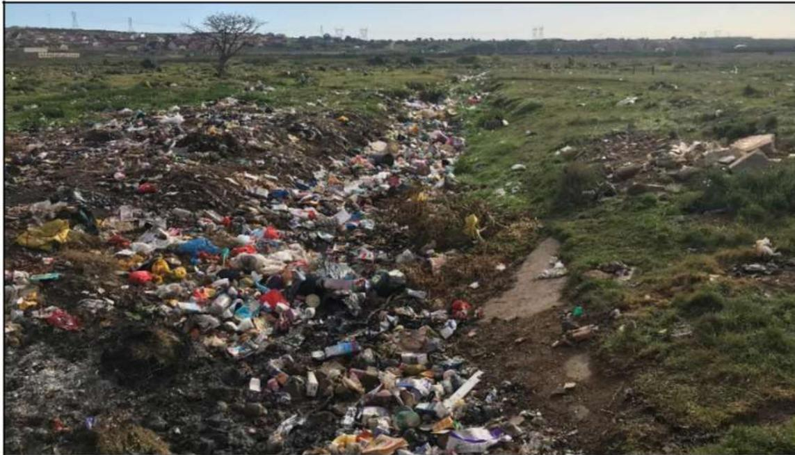
**Figure 4-15** One of the many stormwater canals that conveys stormflows into the Chatty River Wetlands. Many of these canals have been totally blocked by the litter and debris, causing them to overflow into inhabited areas, potentially posing a health risk to those living nearby. In addition, the canalised stormwater conduits that are not blocked were observed to, in some cases, have resulted in erosion and scour of the downstream wetland.
