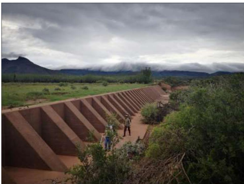
**Figure 4-31** View of a buttress weir and the upstream wetland and grazing areas
