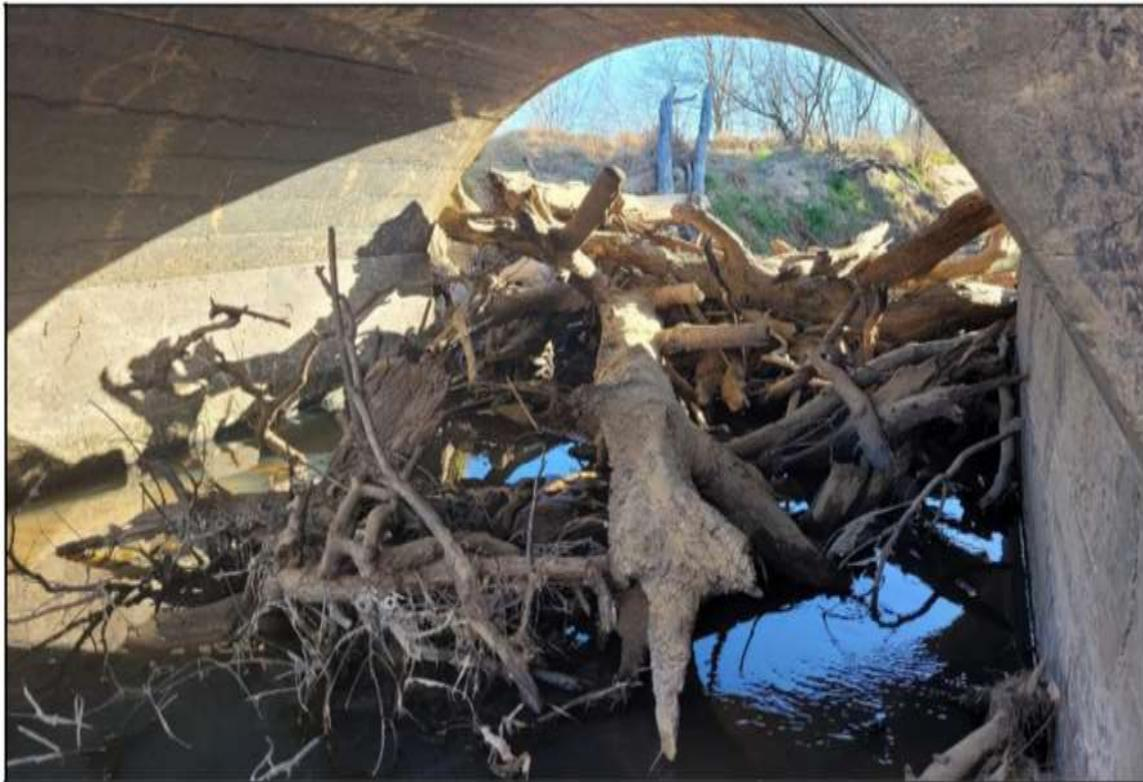
**Figure 4-52** Debris below a large road culvert across the incised portion of the floodplain.
